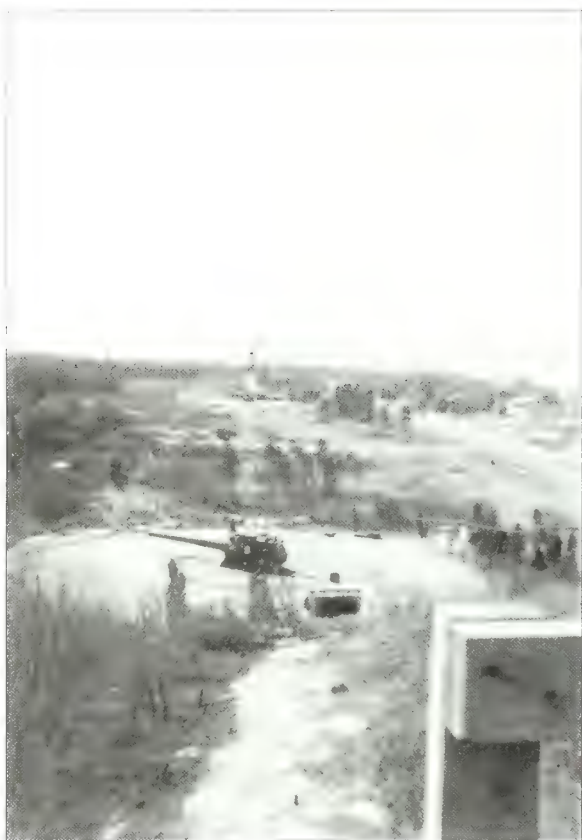
Figure 2.43. View looking south at emplacement #1, Battery Kingman, circa 1940–41. In 1919, both Batteries Kingman and Mills were armed with twelve-inch guns that had no concealment or protection from above. The guns were mounted on high-angle carriages set on rotating platforms that resulted in a 360-degree field of fire. Battery Mills' emplacement #2 and central earthwork can be seen in the background (GATE 938).
